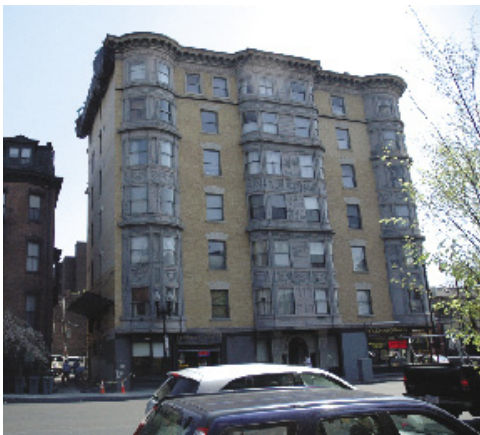
Before restoration - Tremont Towers Condominiums - Boston, MA
