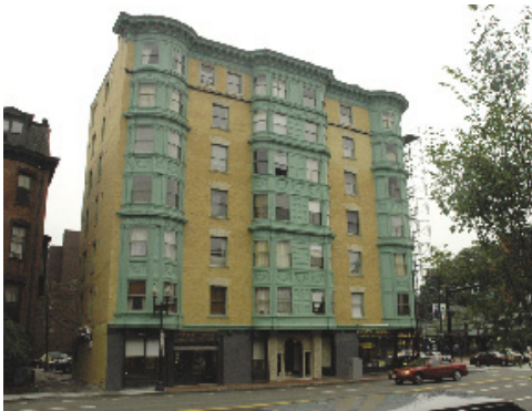
After restoration - Tremont Towers Condominiums - Boston, MA
